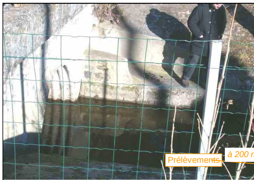
Photo aval de "Pt06"
